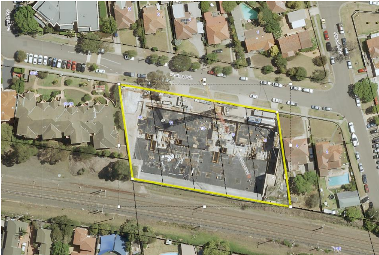
Image A: Aerial View of the Site
